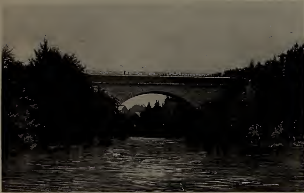
ECHO BRIDGE , Viaduct of the Boston Water Works. Over Charles River, at Hemlock Gorge Reservation of the Metropolitan Park System, suburb of Newton Upper Falls.
